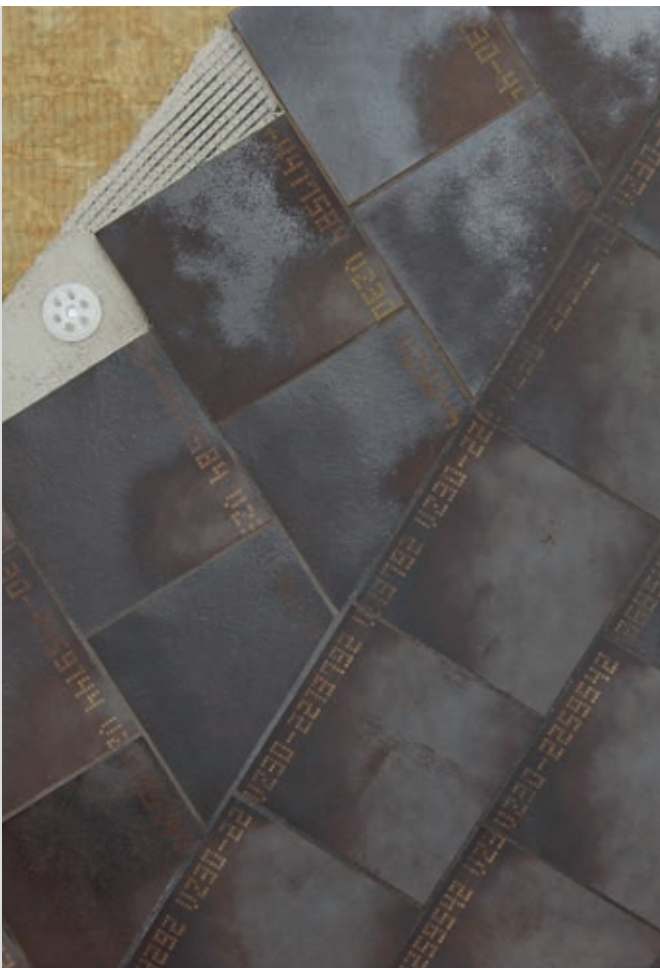
Shuttle facade ceramics on ETIC system
